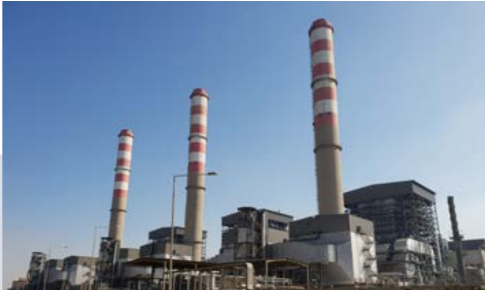
South Helwan UEEPC (EGYPT) SC thermal powerplant 3 x 650 MW Gas/Oil Benson Boilers
