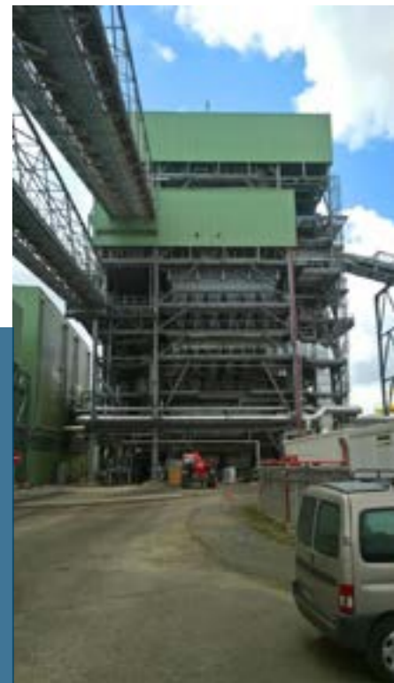
Martinica Albioma (French Overseas Territory) Biomass (wood chips/ wood pellets / bagasse) grate fired boiler 135 t/h steam capacity
