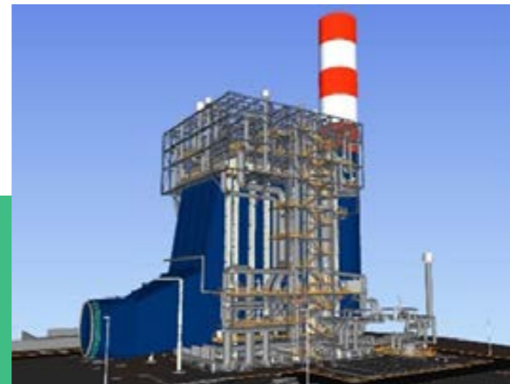
Marghera Combined Cycle AEN for Edison (ITALY) 1 HRSG behind GT36 H class 500 MW GT
