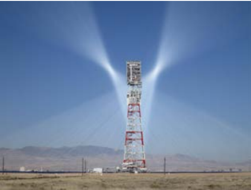
Coalinga (California) Solar receiver for Concentrated Solar Power tower type plant
