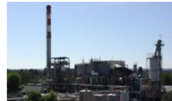
CCA facility – 49 MWth test rig
