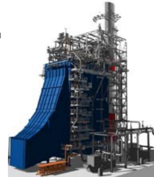
Mirfa Combined Cycle ADWEA (Abu Dhabi- UAE) 3 HRSG with supplementary firing behind F class GT
