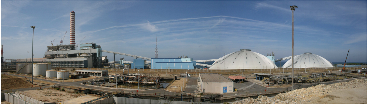
Fig. 2 - Torrevaldaliga North Power Plant view including coal handling systems and Storage domes
