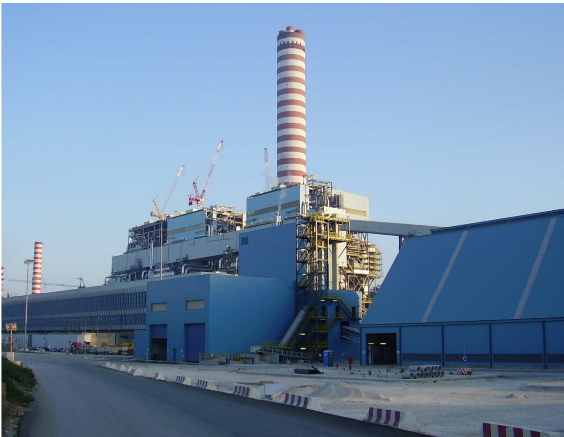
Fig. 1 - Torrevaldaliga North Boilers view
