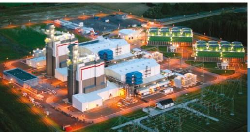
Hamm Uentrop Trianel (GERMANY) 2 HRSG behind 2 x 250 MW GT
