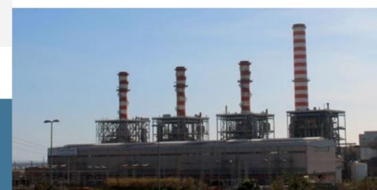
Torrevaldaliga South Combined Cycle Tirreno Power (Italy) ITALY 3 HRSG behind 3 x 250 MW GT
