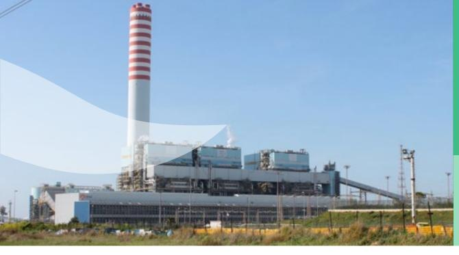
Torrevaldaliga North Enel (ITALY) USC Coal Fired Benson Boiler 3 x 660 MW, 252 bar, 604/612 °C
